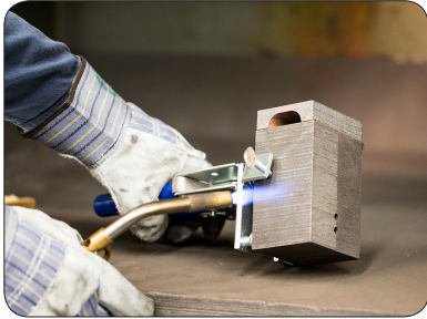
Step 1: Torch dry the mold before making the first connection.
