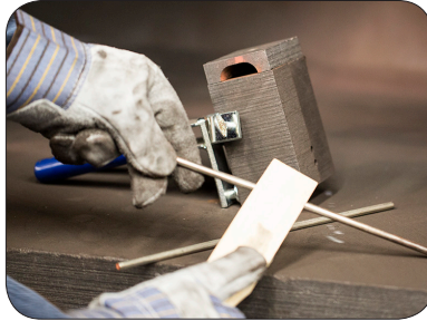
Step 2: Clean and dry conductors, insert conductor into mold, close handle clamp and lock mold.
